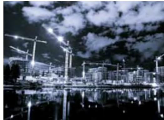
Athletes Village construction in Vancouver, BC
